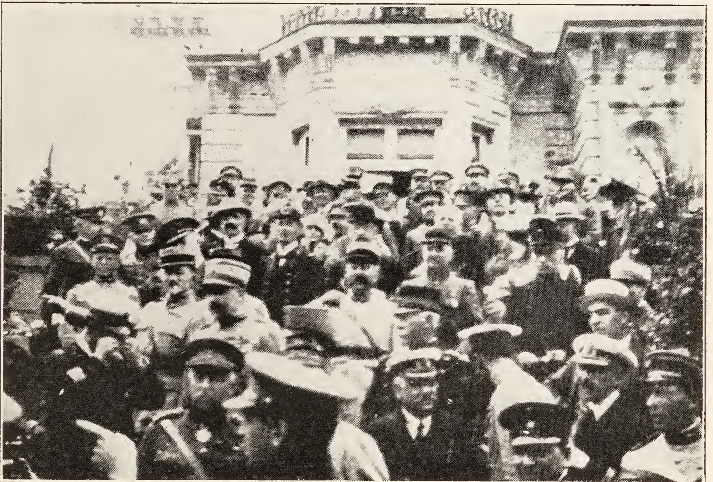
SPA. AFTER AN INSPECTION OF THE HYDRO:
